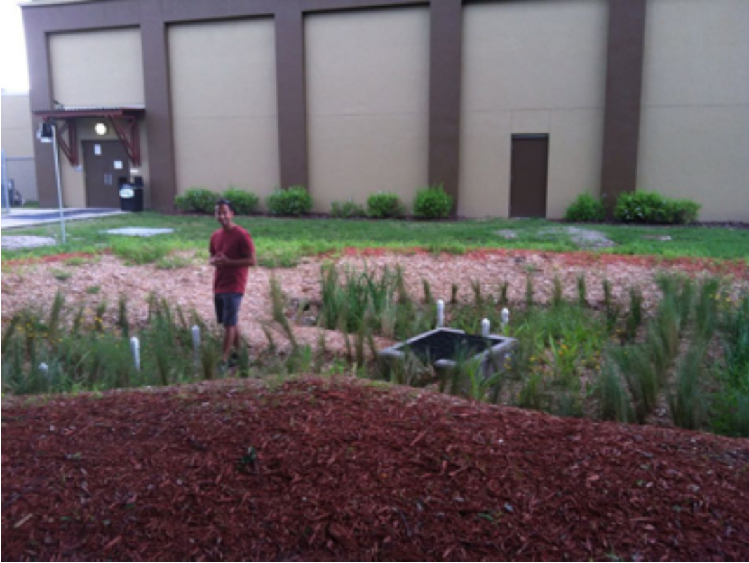
Figure 3: Rain garden with weather station constructed on the property at Young Middle Magnet for stormwater management.
